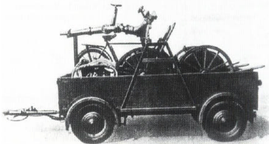
Right: 0.75-ton A 2 Standard Trailer as hose reel trailer for the 1936 and 1941 model hose trucks (Kfz.346). The trailer's load consisted of 8 B-Type pressure hoses on wheeled reels, 22 C-Type pressure hoses on wheeled reels, 1 bicycle, 1 inflatable boat, 1 swivelling nozzle holder. (L.Dv.783/3 + 783/3a)
