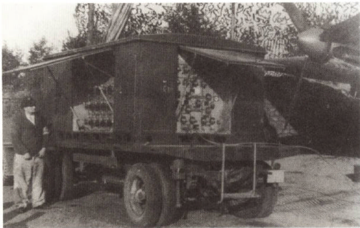
Two-axle trailer with special body for filling the oxygen systems of combat aircraft.
