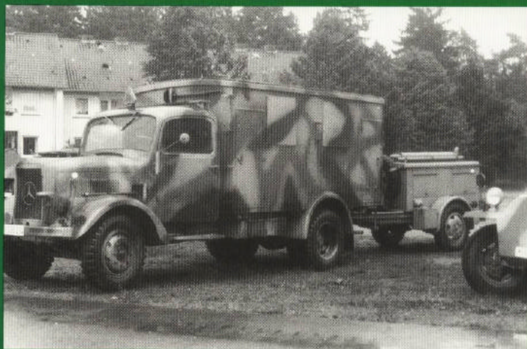
This heavy Type-A field generator unit (SdAh.24) was displayed at the Bundeswehr's Combat Forces School II at Munster on "Armored Fighting Forces Day." The trailer was pulled by a Mercedes-Benz L 3000 S radio truck.
